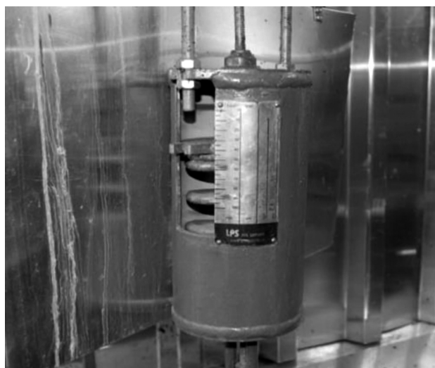
Figure 3: Spring support of the transition pipe Slika 3: Vzmet v pretočni cevi
