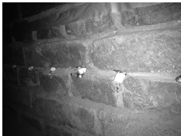
Figure 2: Drill holes filled by waterproofing gel
