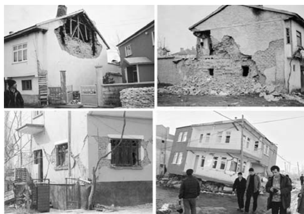
Figure 1: Some damaged masonry buildings 14 (Sultandagi-Cay Earthquake, 2002)
